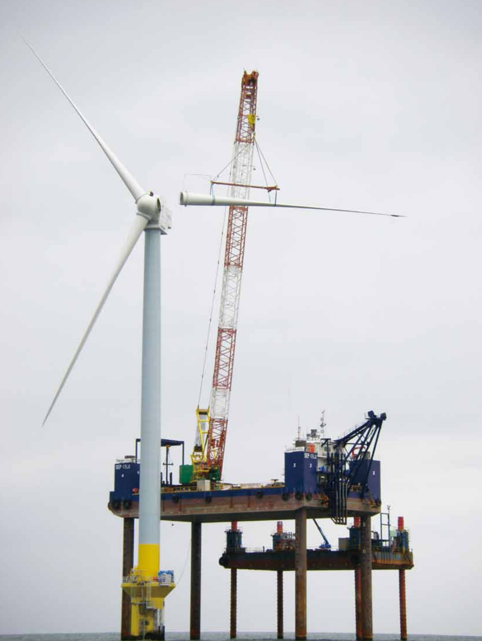
Installation of the offshore wind turbine (offshore Choshi), October 2012
