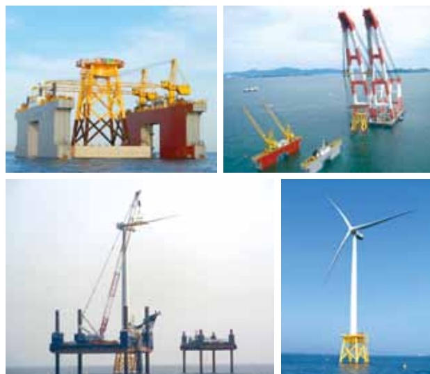
▲ From the left: Shusaku Nakashima and Yutaka Yoshimura of Electric Power Development Co.; Sumihisa Kozono and Noboru Matsumoto of Penta-Ocean Construction Co. ▶ Installation of the hybrid gravity type substructure and the offshore wind turbine.
