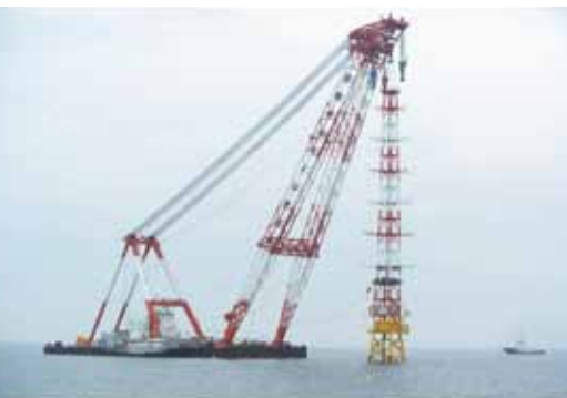
▲ Installation of the wind condition observation tower (offshore Kitakyushu City)
