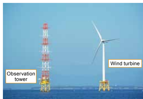
▲ Wind condition observation tower and wind turbine offshore Kitakyushu City (Fukuoka Prefecture)
