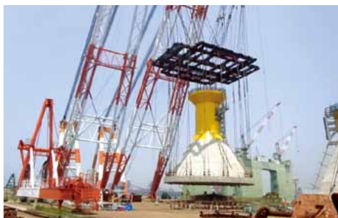
The completed foundation was loaded onto a floating dock and transported, then lowered from a crane barge for installation at the prescribed location.
