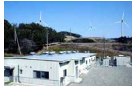
Wind turbine generator
