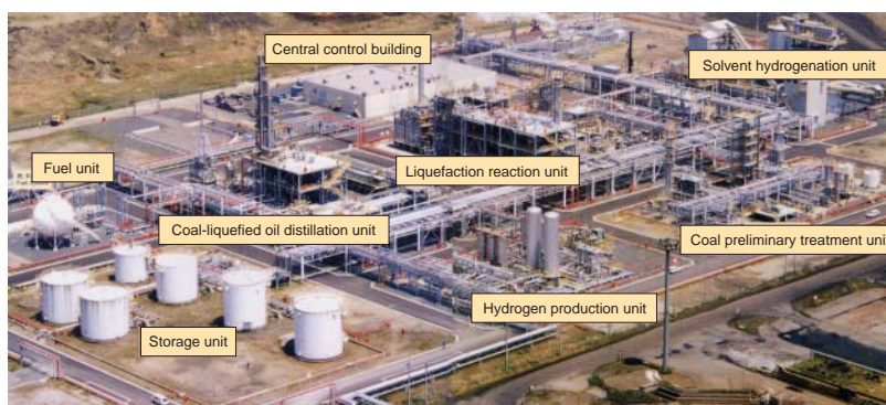
Fig. 3 Total view of NEDOL Process pilot plant (150 t/d)
