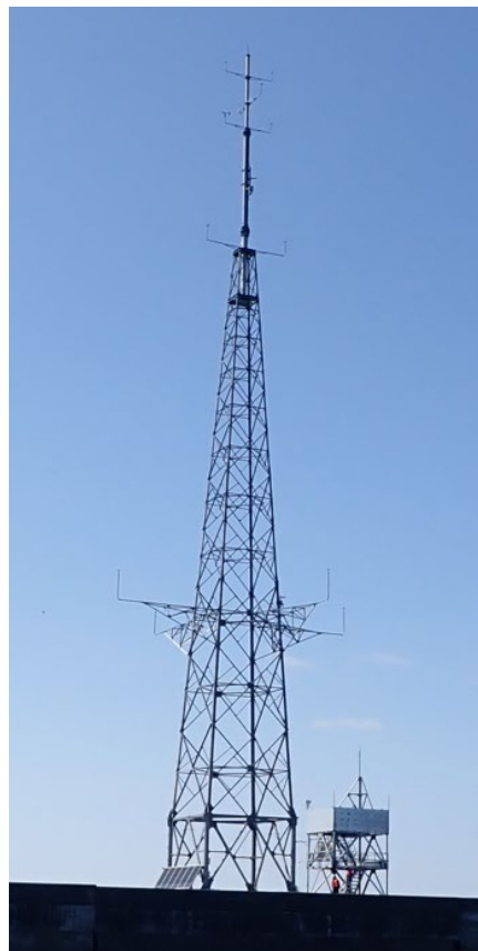
Figure 3.2 Example of offshore meteorological mast (Mutsu Ogawara Port)
