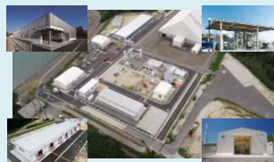
R&D and Demonstration Base for Carbon Recycling
