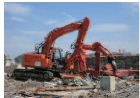
Metal scraps from construction structures and foundations complicatedly intertwined with each other were finely cut and separated to be transported. (Minami-Sanrikucho)
