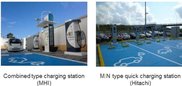
Figure 2 2 types of quick charging station
