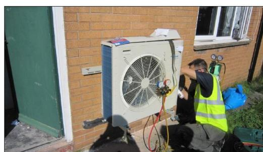
Figure 7 Installation of outdoor unit
