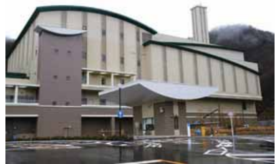
Kunisaki Clean Center, the first facility to install the Hyper 21 Stoker System Two furnaces are able to treat 235 tons of waste per day. Recovered heat from furnace is used to generate power and heat water.
