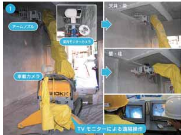
Demonstration for stripping and removing of simulated asbestos
