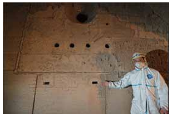
Inner wall of a furnace
