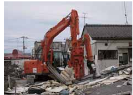
A cargo container drifted by the tsunami and blocking a road in the city was disassembled and separated on the spot to be transported. (Ishinomaki City)
