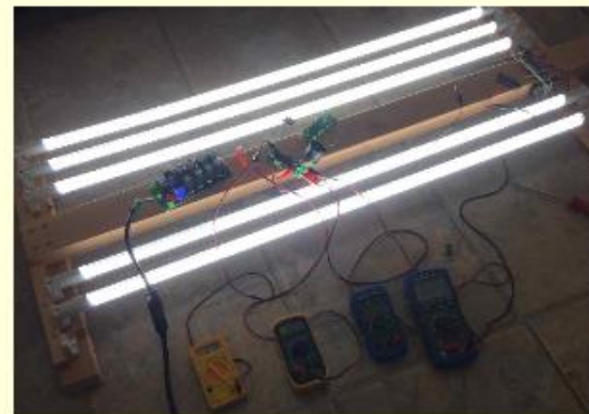
Zone Light, 380 V DC, 6% W saved
