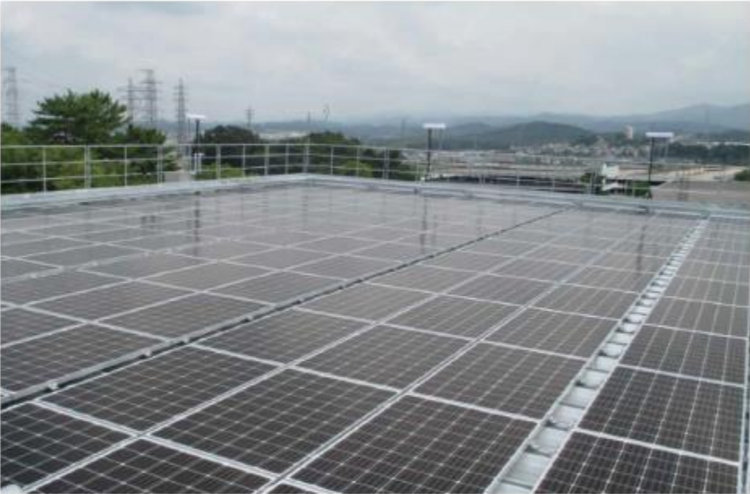
Solar power generation at the plant site
