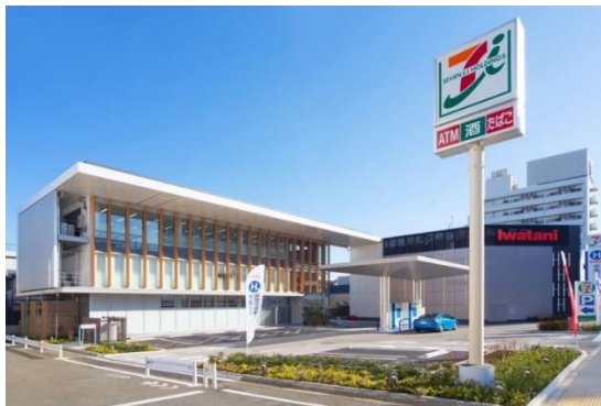
Iwatani Hydrogen Refueling Station in Tokyo Ikegami
