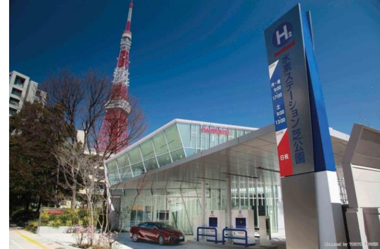
Iwatani Hydrogen Refueling Station in Shibakoen
