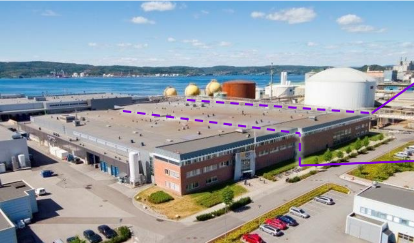
The new manufacturing facilities are located in Herøya Industrial Park, in a 15,000m 2 building in one of the largest industry parks in Norway
