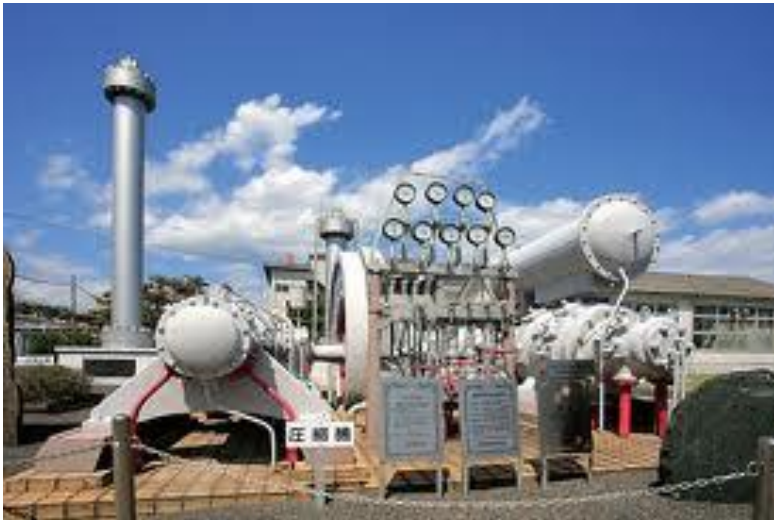
Monument of Casale's High Pressure Ammonia production Plant in Nobeoka city
