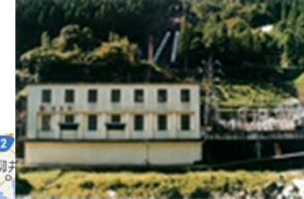
Suigasaki power plant
