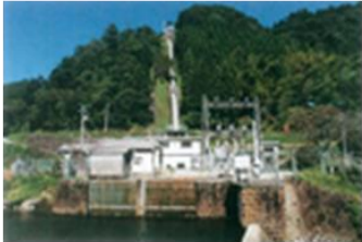
Hakusi power plant
