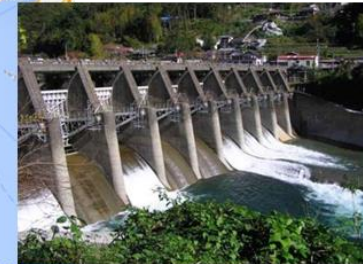
Hoshiyama power plant
