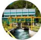
HYDROELECTRIC POWER GENERATION
