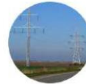
TRANSMISSION GRIDS AND SUBSTATIONS
