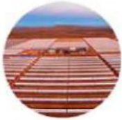
THERMAL POWER GENERATION
