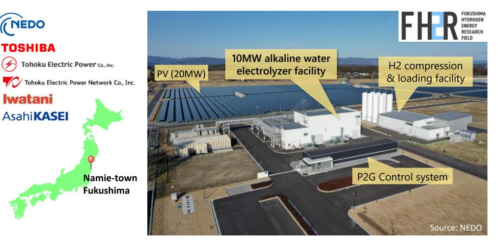
FH2R is a 10MW-class hydrogen production plant with 20MW PV, started in Feb. 2020.
