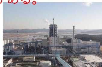
• First 250MW IGCC in China • First 2000t/d Dry Coal Powder Gasifier in China • Design, Construction, Commission and Operation by CHNG
