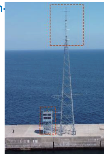
▲Weather observation mast installed on a breakwater at Mutsu-Ogawara Port
