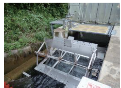
Non-electric garbage remover Source: Aratani Civil Engineering Consultants Co., Ltd.
