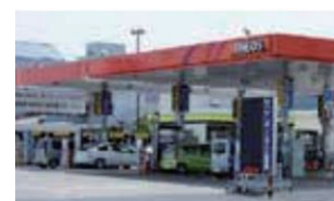
2012 Commercial model demonstration hydrogen station constructed
