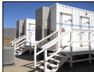
Energy Storage Facilities(Li-ion Batteries and Heat Batteries) Source: NREL and RONDO
