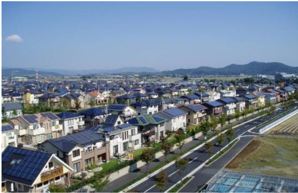
Example of solar power generation in a group of stand-alone houses Total: 2,130 kW, 553 households (3.85 kW/household on average) (Ota City, Gunma Prefecture) Source: Photograph provided by Ota City Land Development Corporation
