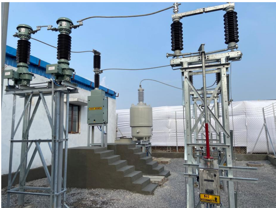
Micro substation with a PVT
