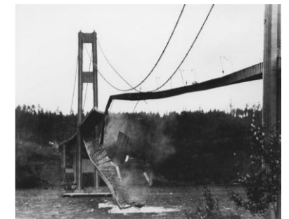
due to strong wind resonance Collapsed Tacoma Bridge (1940)
